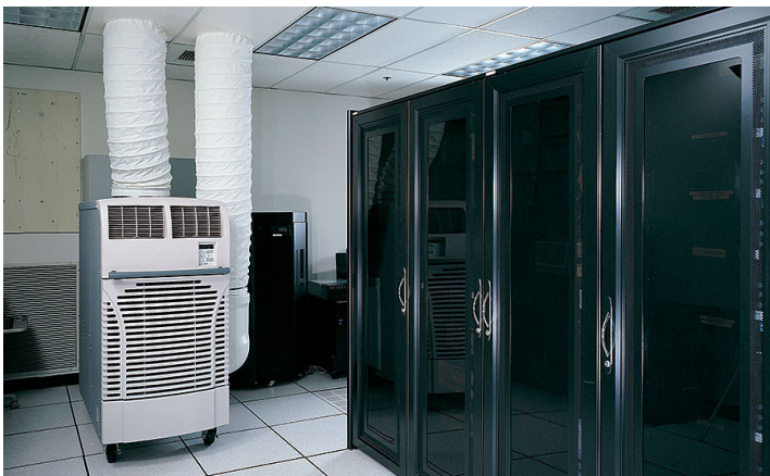
On Demand: Uptime is a significant benefit of portable units, which can be deployed on-site and can be operational within hours of a shutdown event.
